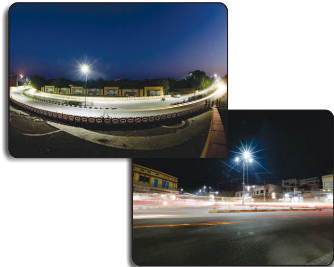
Energy efficient LED Street Lights installed across Rajasthan
